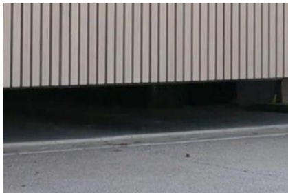
OAK SLAT · SECTIONAL BATTENS RUN THROUGH THE SECTION JOINTS
